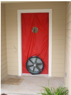
Figure 1. A blower door test set-up on a new home as it appears from the outside of the building.
