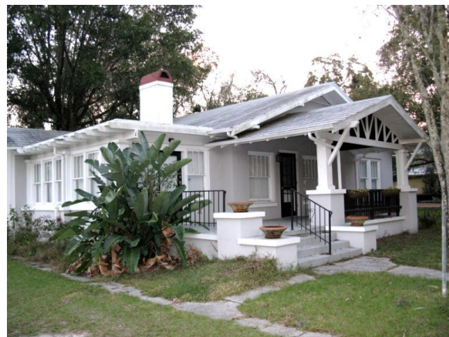
Figure 1. Before: Bungalow Studio prior to building and landscape improvements. (Image Courtesy: Chris Lathrop)
