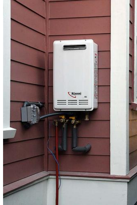
Figures 1 and 2. 1,2 Whole-house tankless water heaters vary in size, capacity, and water flow rates depending on your household needs and the required temperature rise above your local potable water supply. Generally these units are about one foot wide by two feet high by 1 foot deep and weigh 35-80 pounds. Most manufacturers offer both interior and exterior mountable models. When using gas-fired models, direct venting to the outdoors is required. These are but two examples of many units available today.
