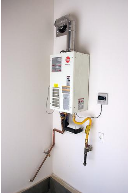
Figures 1 and 2. 1,2 Whole-house tankless water heaters vary in size, capacity, and water flow rates depending on your household needs and the required temperature rise above your local potable water supply. Generally these units are about one foot wide by two feet high by 1 foot deep and weigh 35-80 pounds. Most manufacturers offer both interior and exterior mountable models. When using gas-fired models, direct venting to the outdoors is required. These are but two examples of many units available today.
